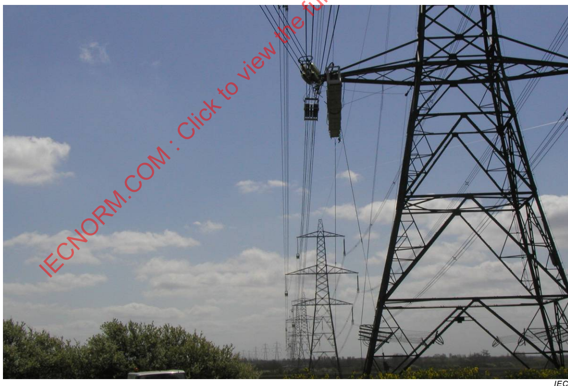
l) Transmission – 2 \times (1 \times n) stringing method
