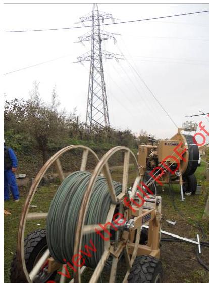
a) Drum puller, two single drums (IEC 60743)
